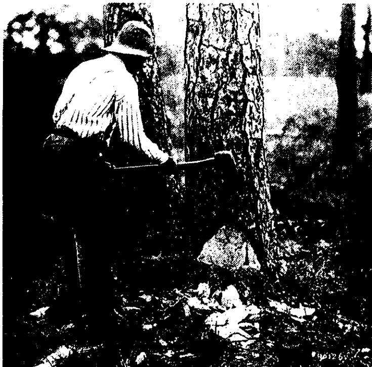
Figure 1. A worker “boxing” the base of a pine tree ca. 1903. The basal cavity will collect resin that exudes from streaks that will eventually be cut at angles into the tree above the cavity (from Butler 1998).
