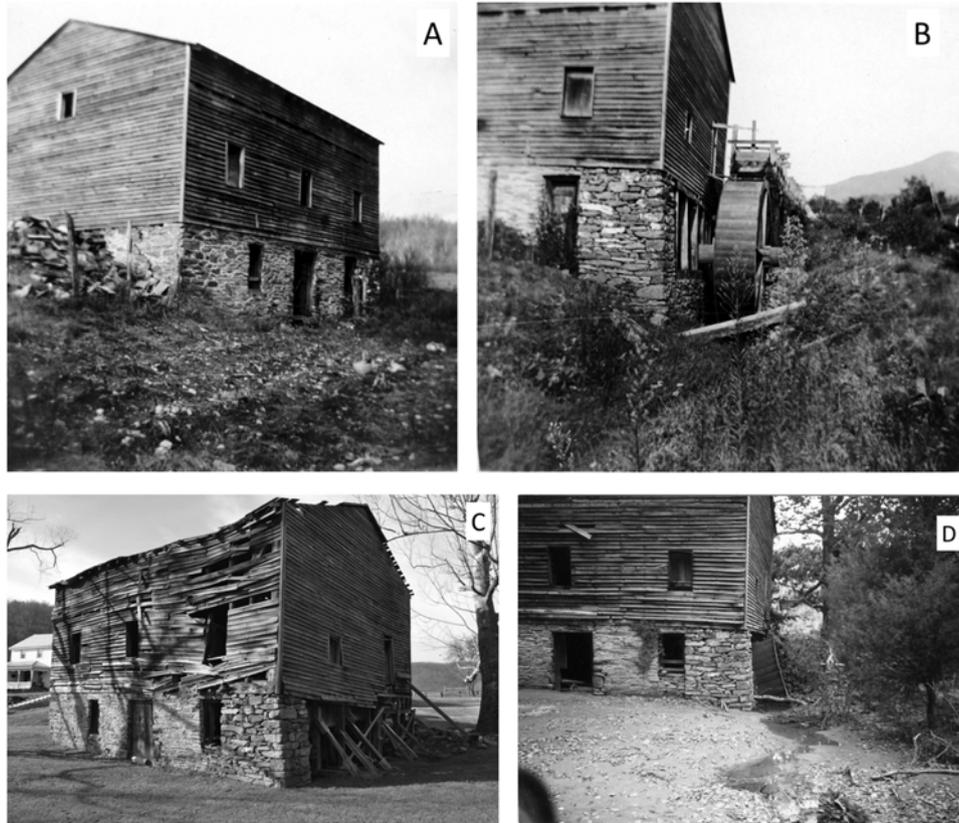
**Fig. 1.** Historical and recent images of the Graves Mill grist mill, located in the Piedmont of Virginia, USA: (A, B) the mill in the 1940s (courtesy Virginia Historical Society); (C) the mill in 2012 (photograph by Douglas Graves); (D) the mill in June 1995 after the June 27 storm, showing deposited sediment around the foundation (photograph by Douglas Graves).
