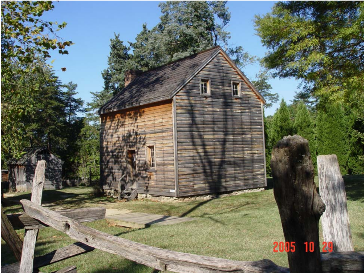
Figure 1. The Joseph Hoskins House, located at Tannenbaum Historic Park, Greensboro, North Carolina. The log structure is currently covered with clapboard siding. The house is believed to date to the Revolutionary War period (ca. 1781), but archaeological testing suggests a later date of construction (Stine 2005).
