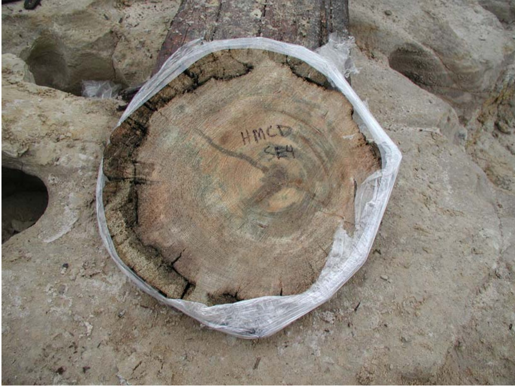
FIGURE 2. Hope Mills crib dam cross section labeled and wrapped for transportation to the Laboratory of Tree-Ring Science.
